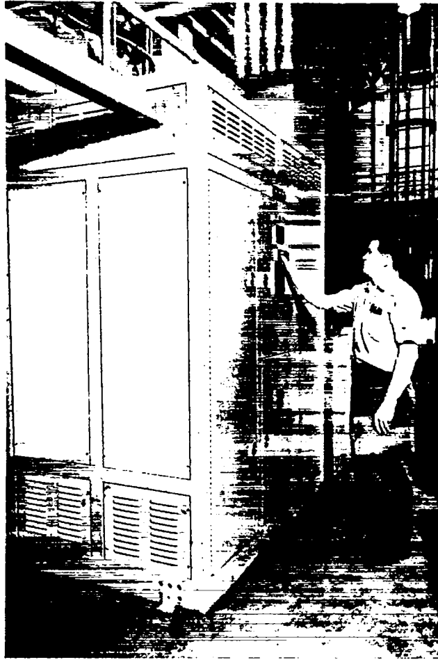
Fig. 11. Power supply installation.
