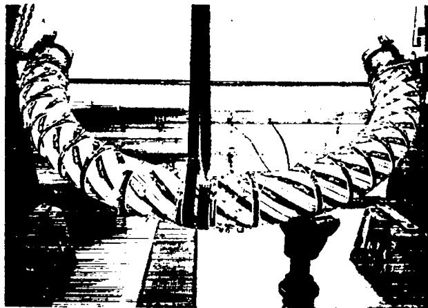
Fig. 4. SF-3C stabilizer conductors.
